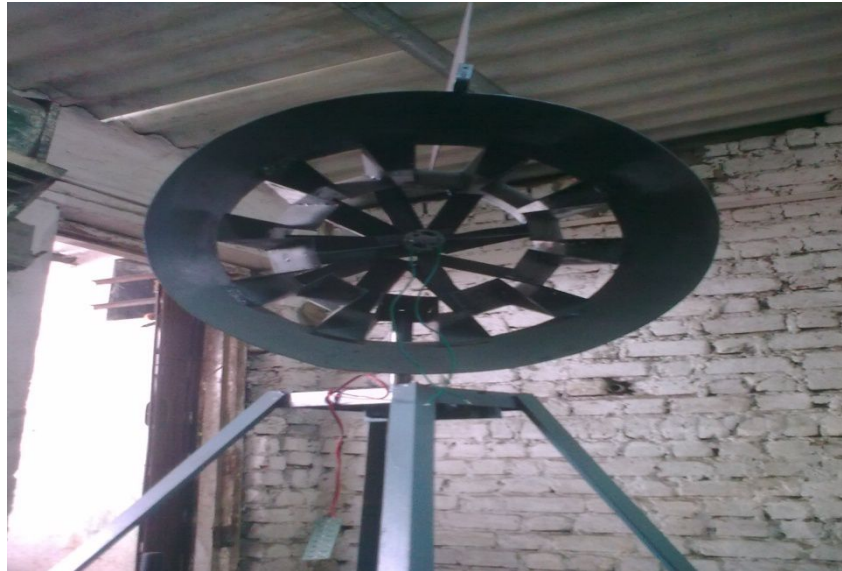
Assembly of jet wind turbine
